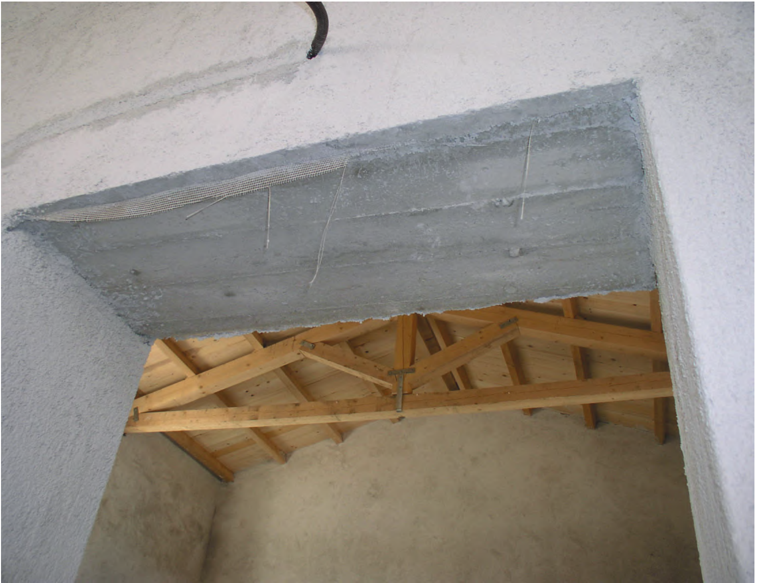
Fig. 61 - Architrave in cemento
